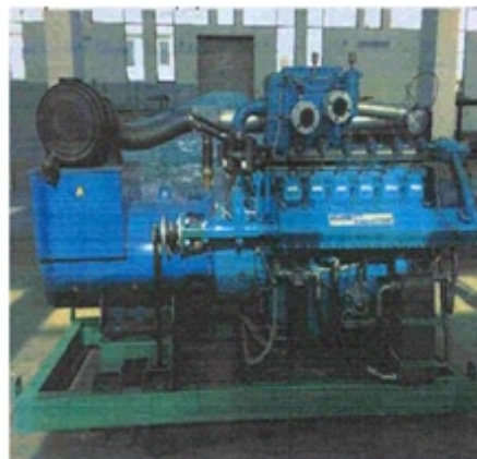
Fig. 4. DG Set, 347 kWe, Schmitt Enertec make
