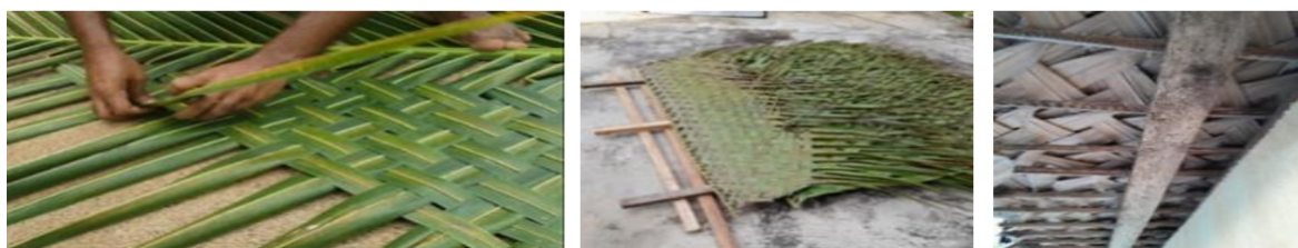
Figure 3. Coconut leaf roof sheets and arrangements
