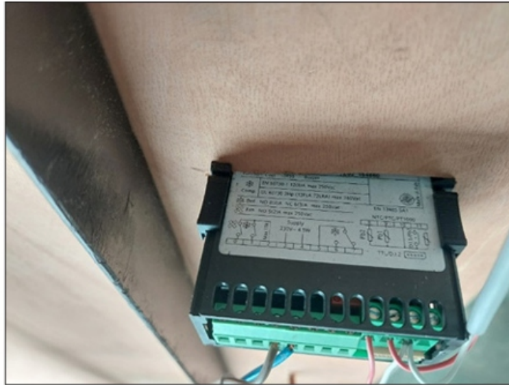
Figure 5. “ELIWELL” IDPlus974 Thermostat Schematic Diagram and Wiring Termination
